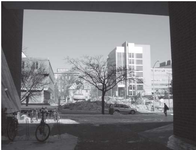
Arrivederci Milan's. A favorite lunch spot for Weeks Hall residents for the past thirty-four years was demolished in December to make room for a six-story 25-unit apartment building (occupancy set for mid-August 2006). Weeks Hall folks currently, and temporarily, have a clear view of the new chemistry building on West Johnson Street (top photo).
